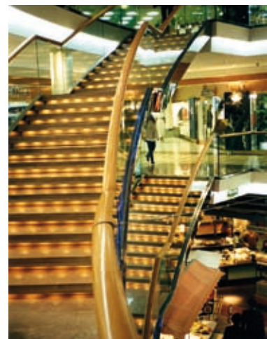
GALLERY , Vienna, Austria Luminaire: AGABEKOV lighting fixtures with Xenon lamps. Same rendering with AGABEKOV lighting fixtures with AGA-LED® lighting units.
