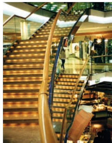
GALLERY , Vienna, Austria Luminaire: AGABEKOV lighting fixtures with Xenon lamps. Same rendering with AGABEKOV lighting fixtures with AGA-LED® lighting units.
